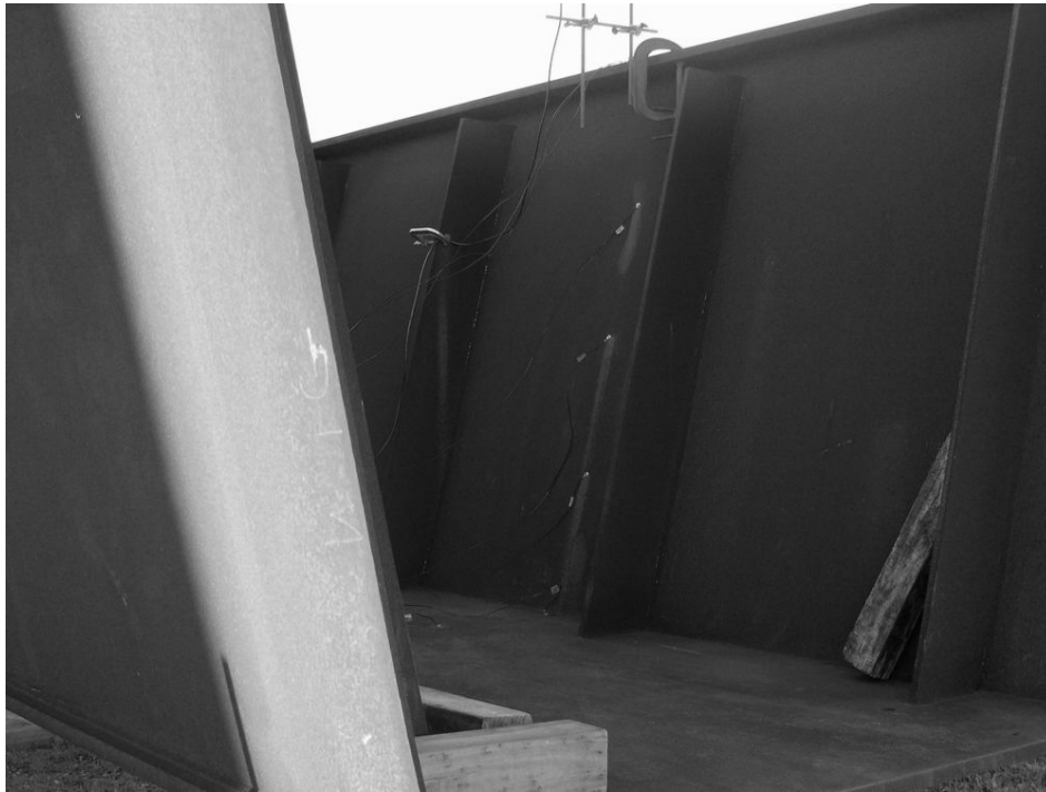
Figure 4.12 Photograph of Morning Sunlight Hitting Eastern Web
