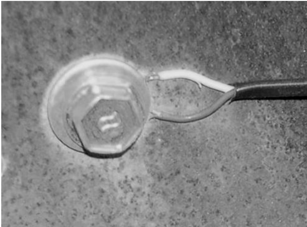
Figure 4.4 Attachment of Thermocouple to Girder Surface
